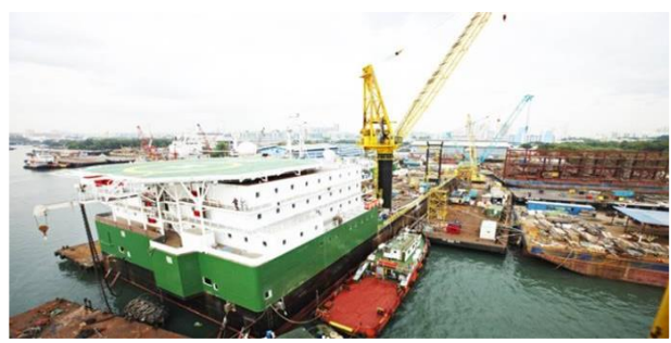
Construction of McDermott LB32 pipelay barge
