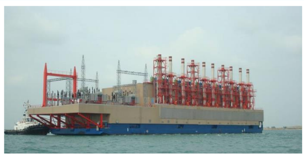
Power Barge Conversion for KPS Alican Bey
