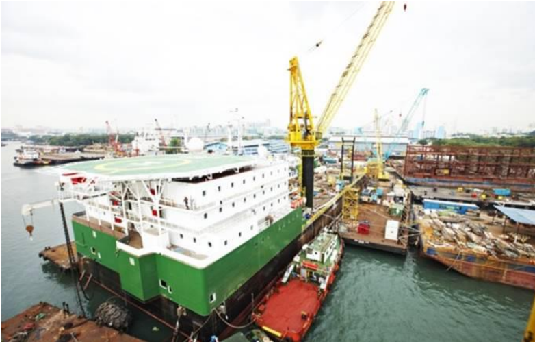
Construction of McDermott LB32 pipelay barge
