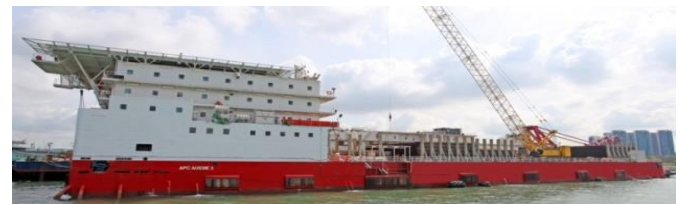
Construction of APC Aussie 1 pipelay barge
