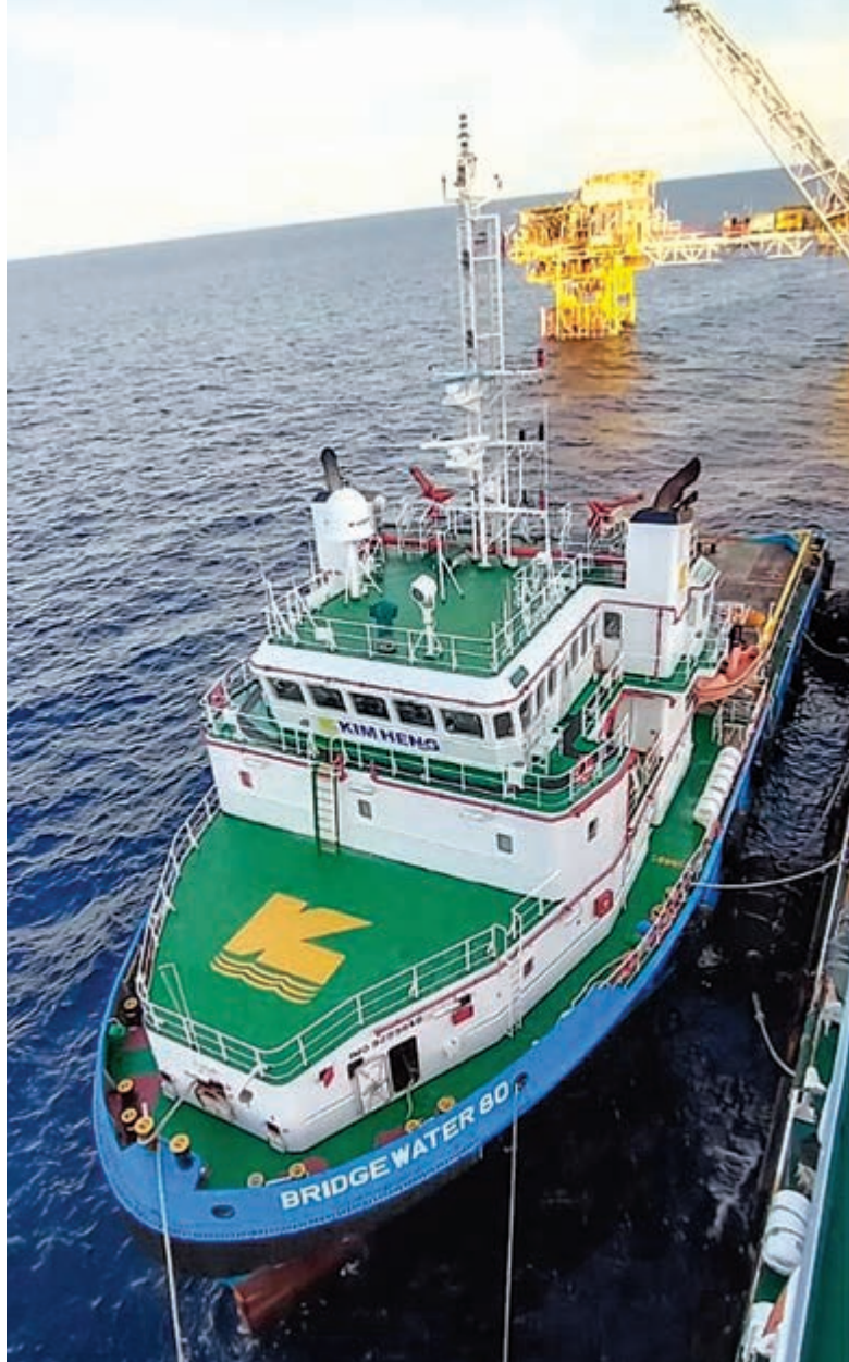
Offshore Platform Works
