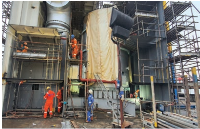
Scrubber Fabrication (Internal)
