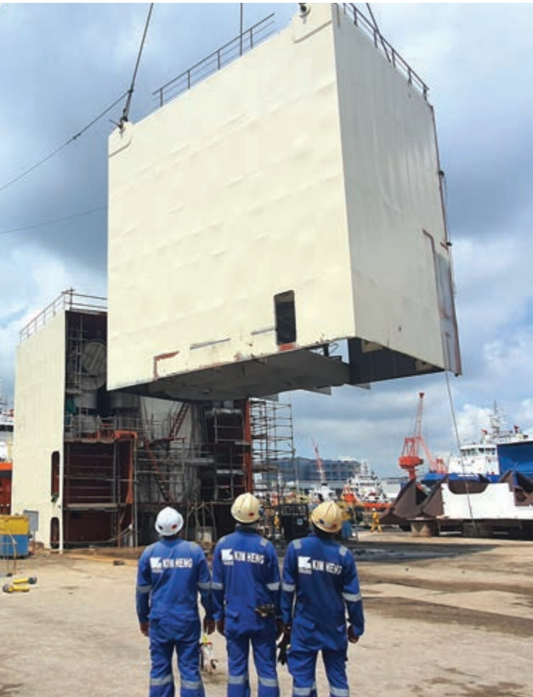
Scrubber Fabrication (External)
