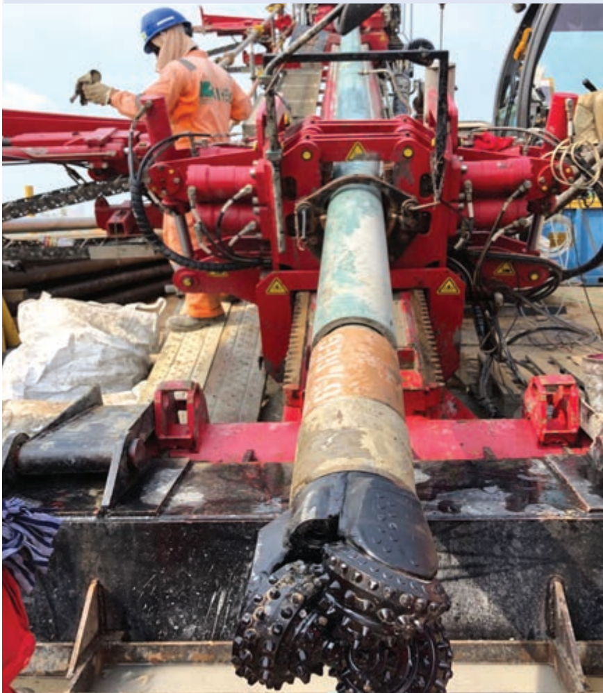
Horizontal Directional Drilling (HDD) Land Rig in Operations
