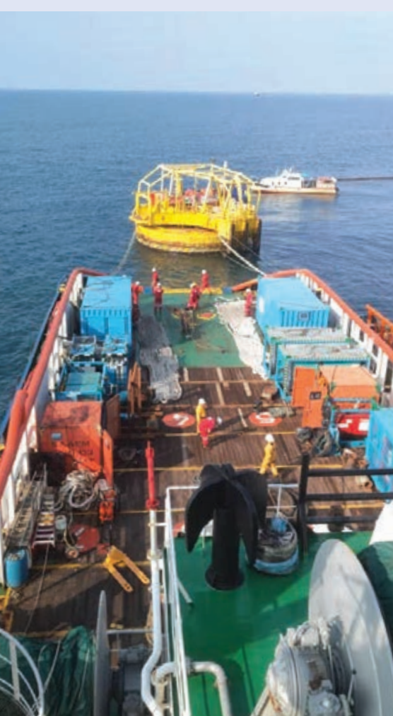
Offshore Buoy Maintenance Works
