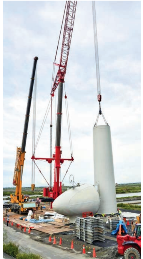
Installation of wind turbine & blade onshore
