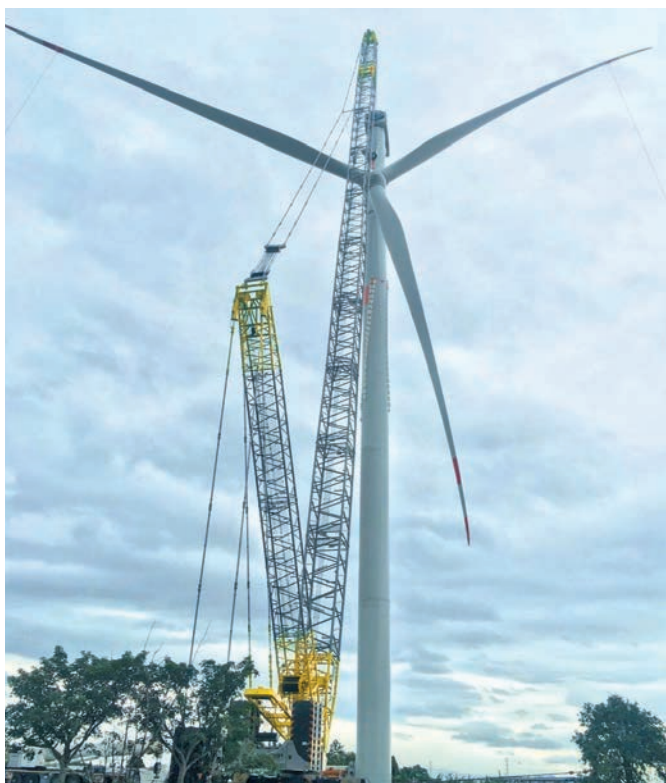
Installation of Wind Turbine
