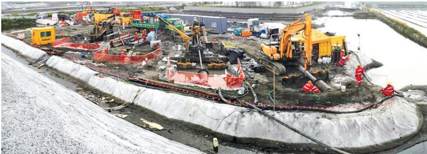
HDD Worksite in Taiwan
