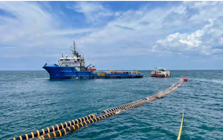
Bridgewater 68 performing Single Point Mooring Buoy repair work in Malaysia
