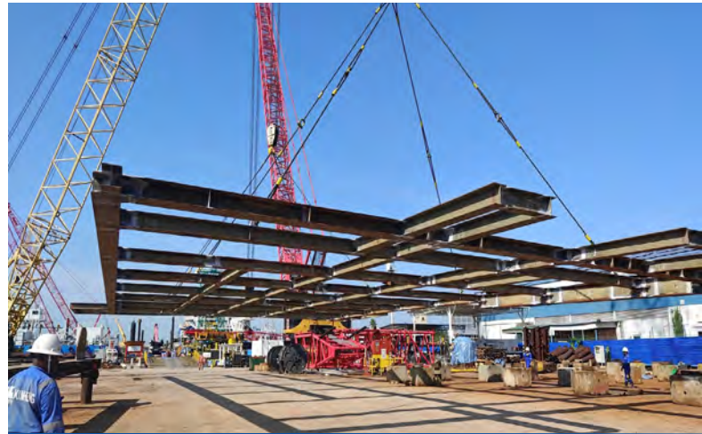
Fabrication of FPSO modules at Kim Heng yard
